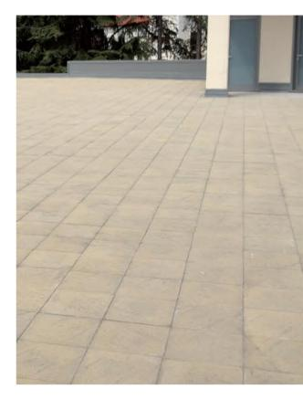
**Panels FRESH HOT application is easy and fast.** In general, they are laid dry directly on the waterproofing mantle, but if some differences in size or not perfectly planar surfaces occur, it's possible to use adjustable-height "little feet" (easy to be found on the market, since they're used for traditional external floor installation), cement compounds for panel fixing and smoothing the surface or shaping the lower part in EPS by yard tools
